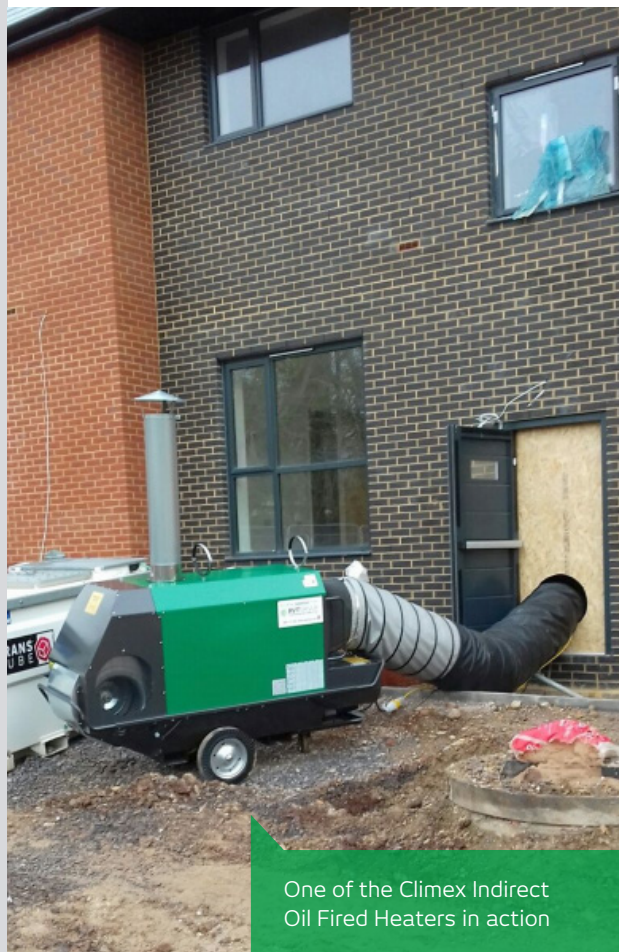
Dry heat was circulated around the building via ducting
