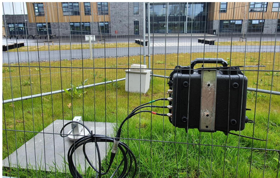
RVT's Monitex® Vibration Monitor On Site.
