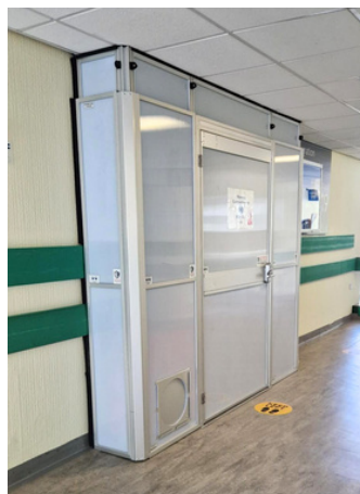
This photo shows the DUSTEX® Aire Guardian Rigid Containment Unit installed between the corridor and the work zone.
