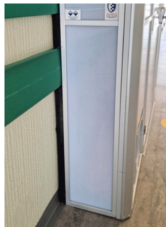
The DUSTEX® Aire Guardian Rigid Containment Unit has a black tight seal around the periphery of the unit to create a seamless barrier.
