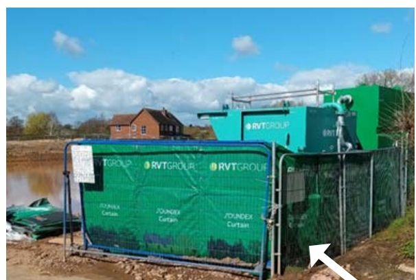
RVT's acoustic curtains are certified to reduce noise by up to 32.9dB and achieve up to 98% noise absorption
