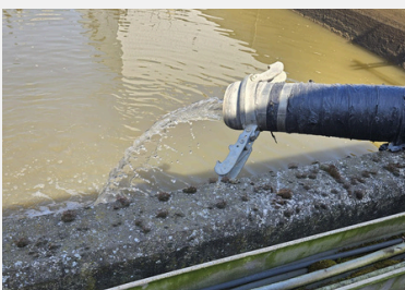
Clean water being discharged in-line with environmental regulations.
