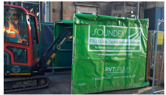
SOUNDEX® Breaker Shroud in use on the project.
