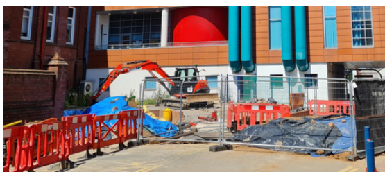
Construction work safely taking place directly outside of the Children's hospital.
