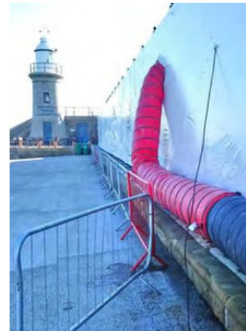
The indirect oil fired heater forces warm air along the ducting, into the sealed building, where it can be evenly distributed using air distribution kits.
