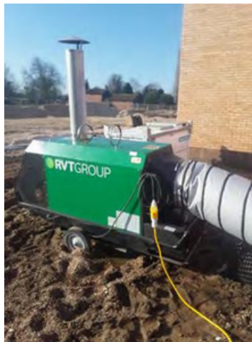
The indirect oil fired heater forces warm air along the ducting, into the sealed building, where it can be evenly distributed using air distribution kits.
