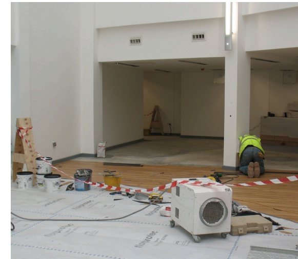
Example of electric heater used to dry out paint work and provide ambient heat whilst other trades continue working.
