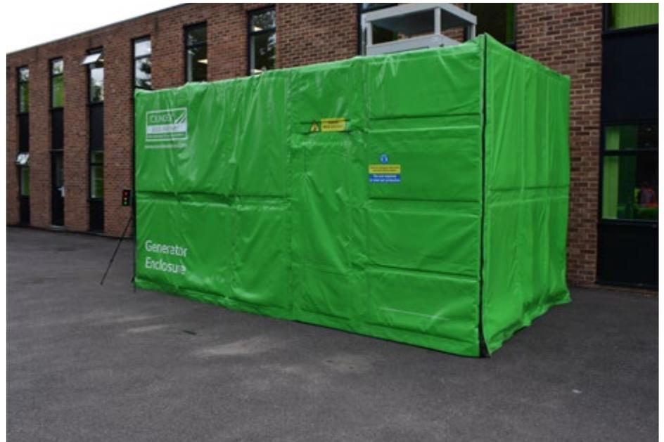
In this picture, a generator has been wrapped by RVT's E3/3 Generator Enclosure. This delivers noise attenuation of between 14.9dB at 50Hz to 59.9dB at 5000Hz. In addition, an A2/3 Soundex Exhaust attenuator sits on top of the generator to subdue noise from the exhaust outlet.
