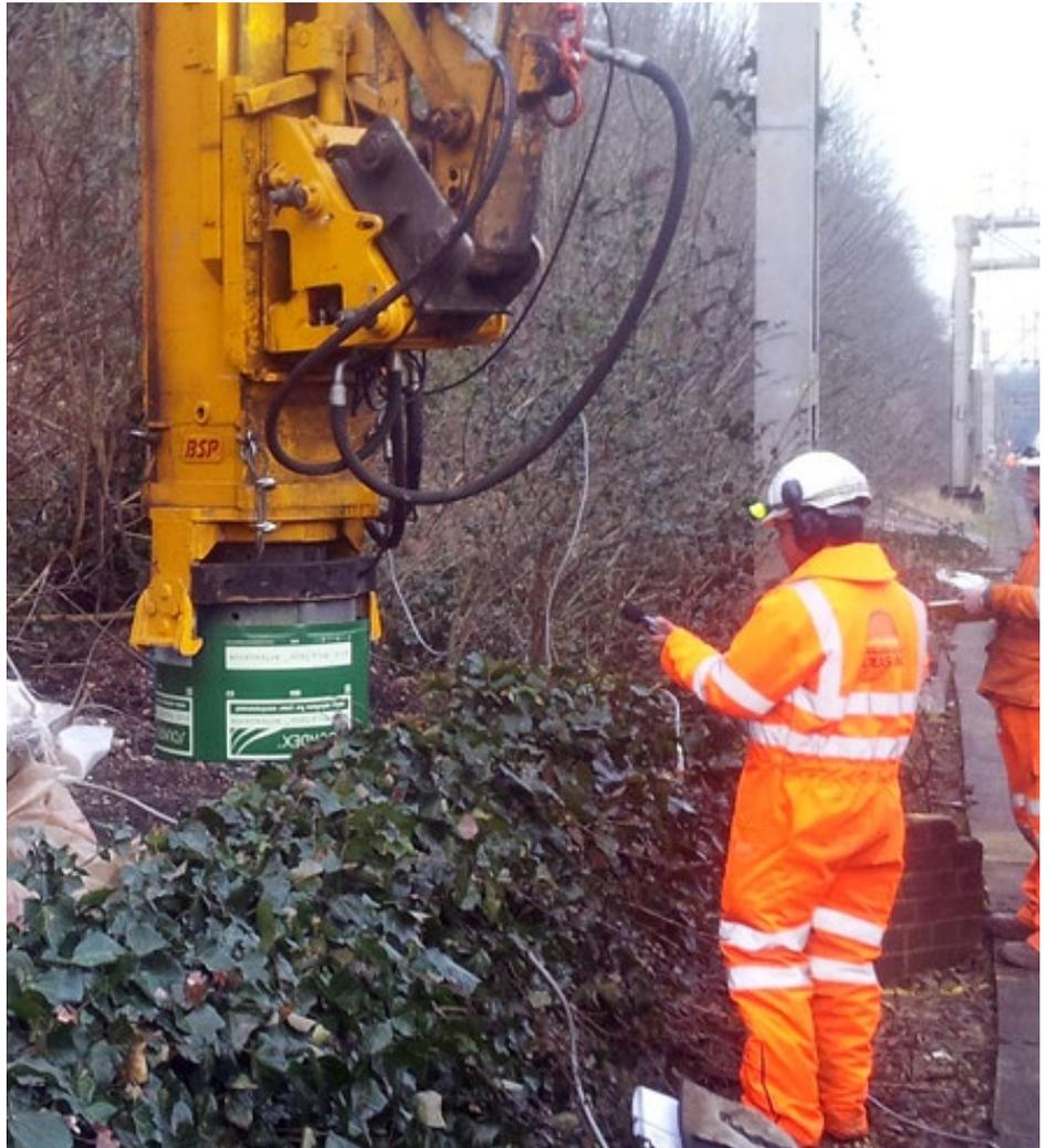
This picture shows RVT's A1/3 Piling attenuator wrapped around the section of pile. Each unit wraps a half metre section of pile, held to it by extra strong magnets. As the pile is driven into the ground the separate attenuators, which are held together by Velcro connectors, can easily be removed.
