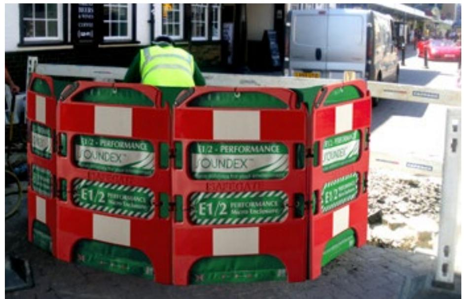
Control measures, such as the noise enclosure above, can be used to significantly reduce noise for those in the vicinity of works being carried out, who are not wearing personal noise protection equipment.
