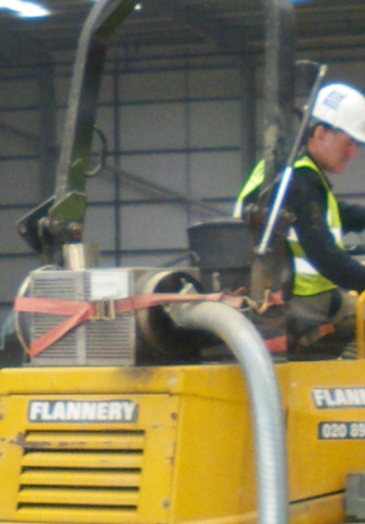
Image above of a diesel particulate filter.
