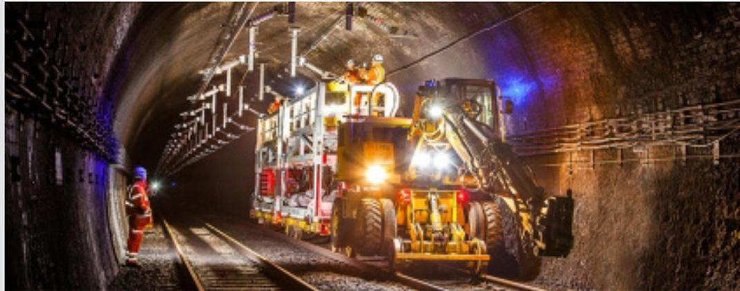
As part of the electrification of the Great Western mainline, a solid overhead conductor rail system needed to be installed in the four kilometre Chipping Sodbury Tunnel. The two conductor rails – one above each track – would provide the power for trains to pass through once the line was electrified.
