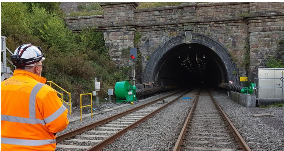
Work in the tunnel proceeded in two phases. During the first phase, from 8 May to 19 July 2017, work proceeded at night using a custom-made rig to drill 4,064 holes in the tunnel roof. Each hole was then fitted with an anchor to support the electrical supply cables.
