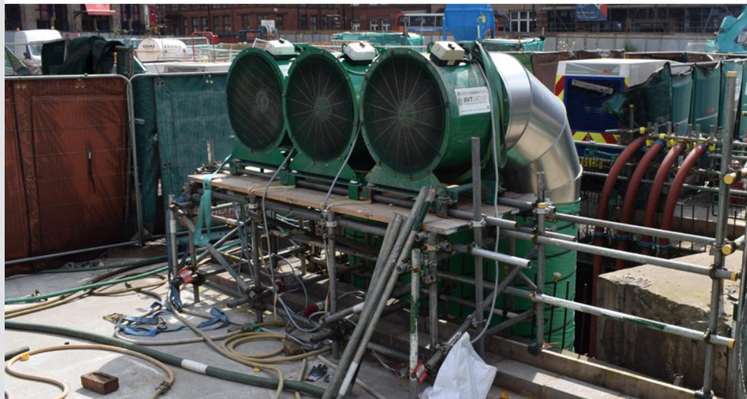
Prior to work starting above ground, extensive hydro-demolition work was required within the existing 4-storey basement. This environment presented challenges in the shape of mist generated by the demolition works and exhaust fumes produced by the diesel plant used. For the demolition workers to operate in safety, suitable counter measures had to be put in place to counter both these hazards.
