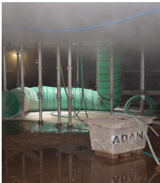
Each individual fan delivers tens of thousands of cubic metres of fresh air every hour and creates a positive pressure to ensure good air quality is maintained. The ducting used to convey the fresh air was strategically routed to provide a safe working environment on each basement level.
